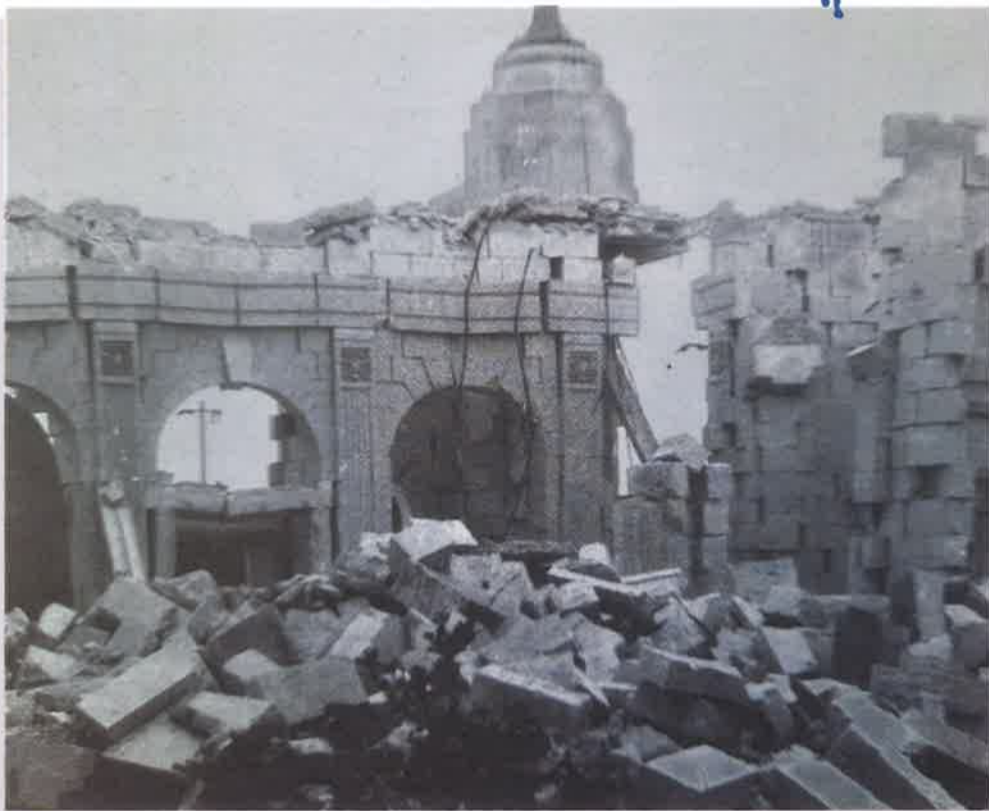
Part of the damaged done during the April 27, 1942 bombing attack
